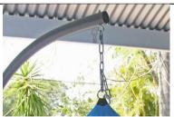
7. From the eyelet, you'll connect a carabiner, then a chain, then finally a carabiner can be hung from a link on the chain depending on how low you want the swing to hang. Then you can connect your swing to the carabiner.
